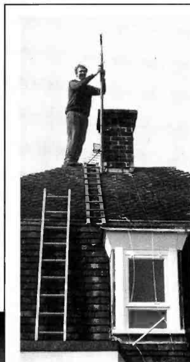
Fig. 1: On his way to the top of his profession! Peter Dodd G3LDO preparing to erect the BWD1.8-30 antenna on the stub mast on his QTH chimney.
