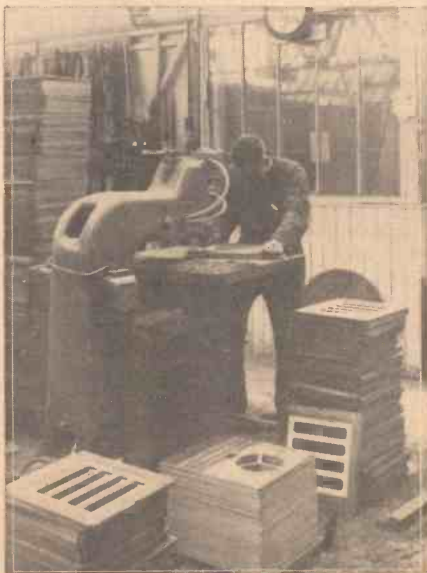
Fig. 2.—Cabinet frets by the thousand are produced in a fraction of the time taken by the old fretsawing method.
