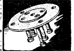
A new Clix chassis-mounting type valve-holder.
